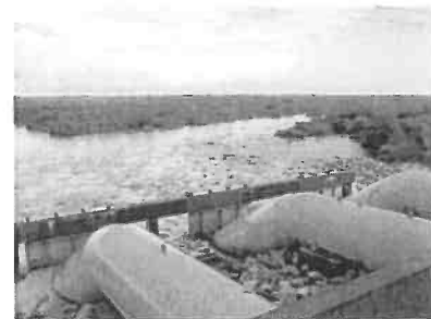
Pump Station discharge into central wetlands
